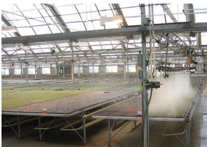
Figure 1. Retractable shade curtains, supplemental lighting, boom misting, and other types of greenhouse equipment can greatly improve propagation of seedlings and cuttings.
